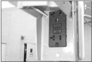
Figure 4.7—Electrical Power Outlet
